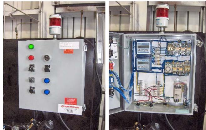
Truck assembly plant coolant proportioning & blending system. Concentrate coolant is pumped from an outside tank to a Pro/Mark PVF-7A proportioner. The concentrate is blended through the proportioner and transferred into an agitated blending tank. From the blending tank, the mixed coolant is pumped out to fill stations on the production line. Project included system design, supply and installation of control, pump station, processor controlled proportioner, turn key installation.
